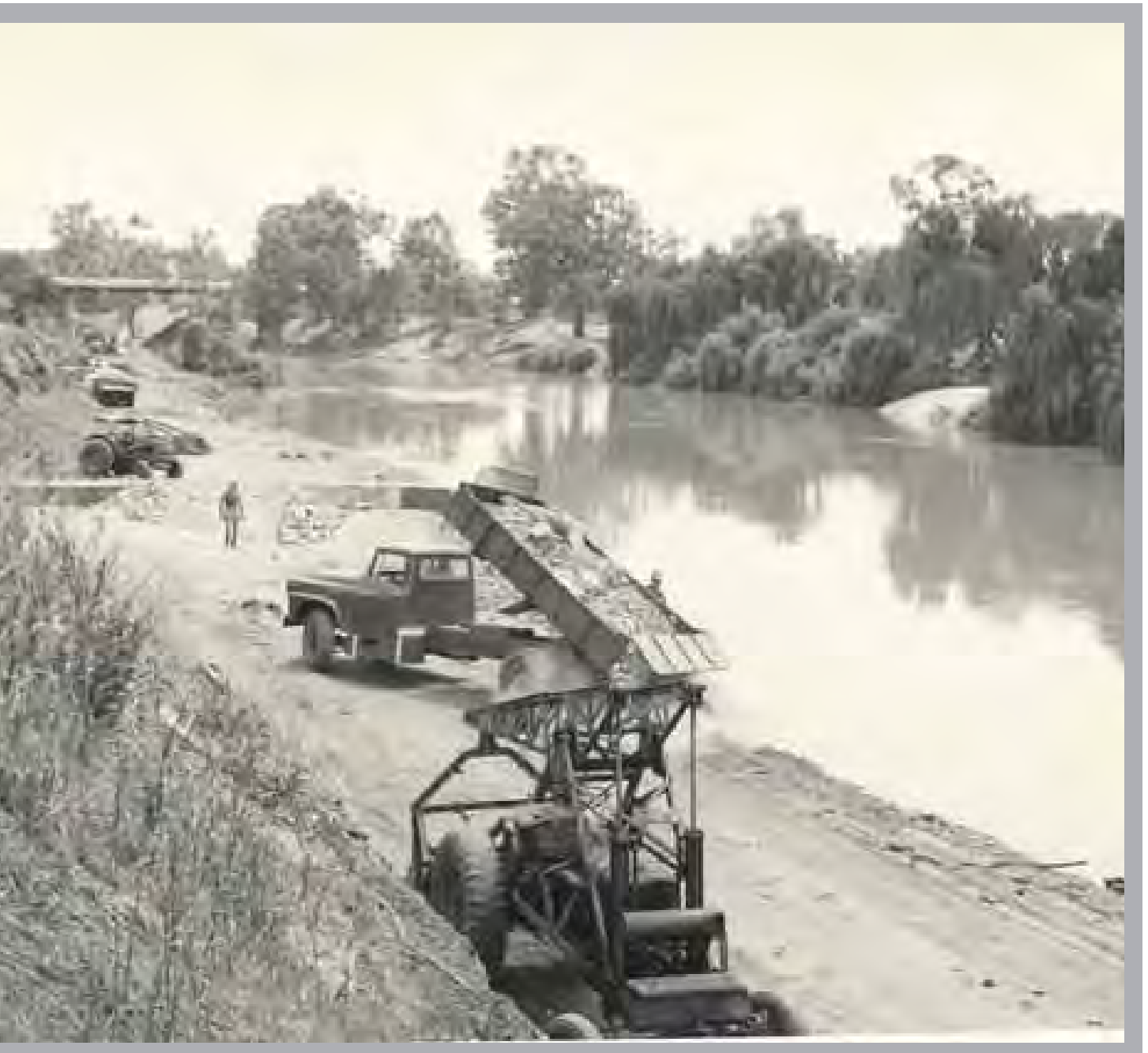
Construction of levee behind Fitzmaurice Street c 1960
