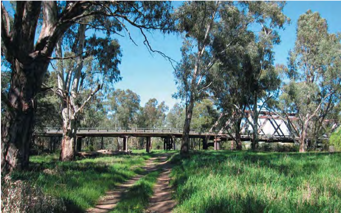
Existing view towards Hampden Bridge
