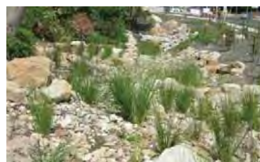
Examples of infiltration area/bio-filter in rock mulch (above) and vegetated swale in median to intercept and clean stormwater. (right)
