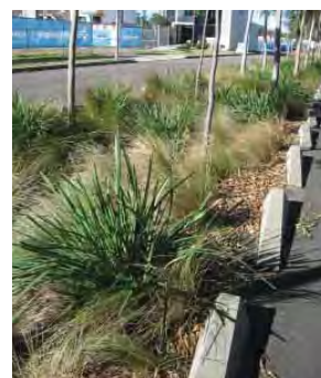
Examples of infiltration area/bio-filter in rock mulch (above) and vegetated swale in median to intercept and clean stormwater. (right)
