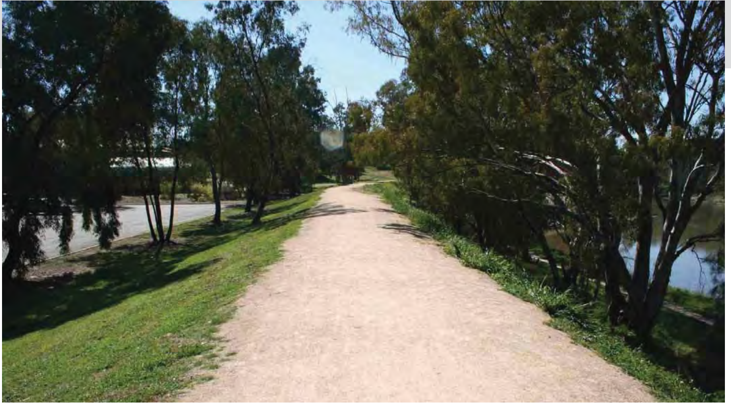
Existing situation of the levee nearby the Visitor's Centre
