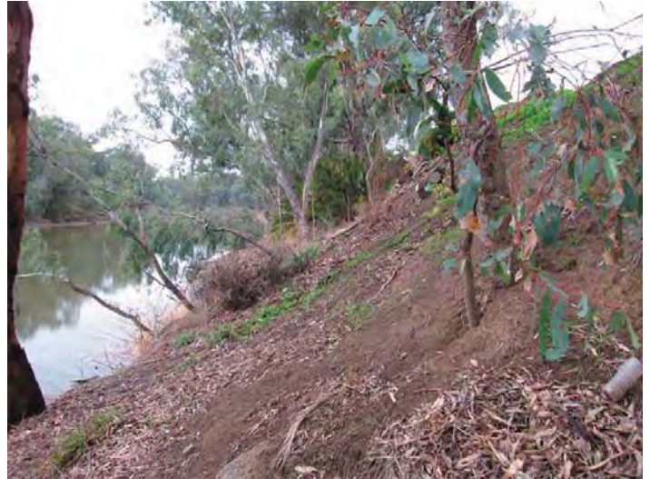
Above: Typical steep banks to the river - northern section of The Bend of the river, where mature trees are falling into the river due to eroding and under-cutting of the banks.
