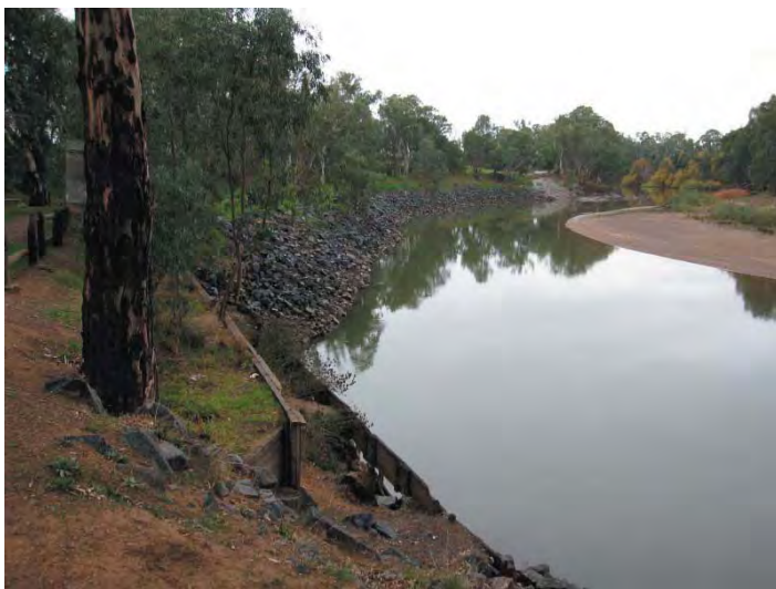
Above: An example of the steep banks with large riprap boulders to the outside of bends.
