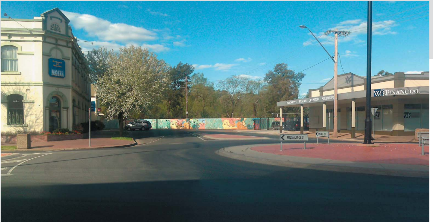
Original levee situation at Cadell Place
